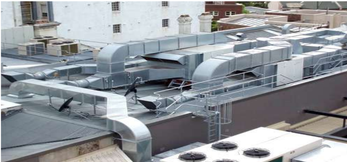
AC DUCTING FABRICATION
