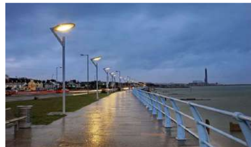
POWDER COATED ALUMINUM HANDRAILS NEAR WATER FRONT
